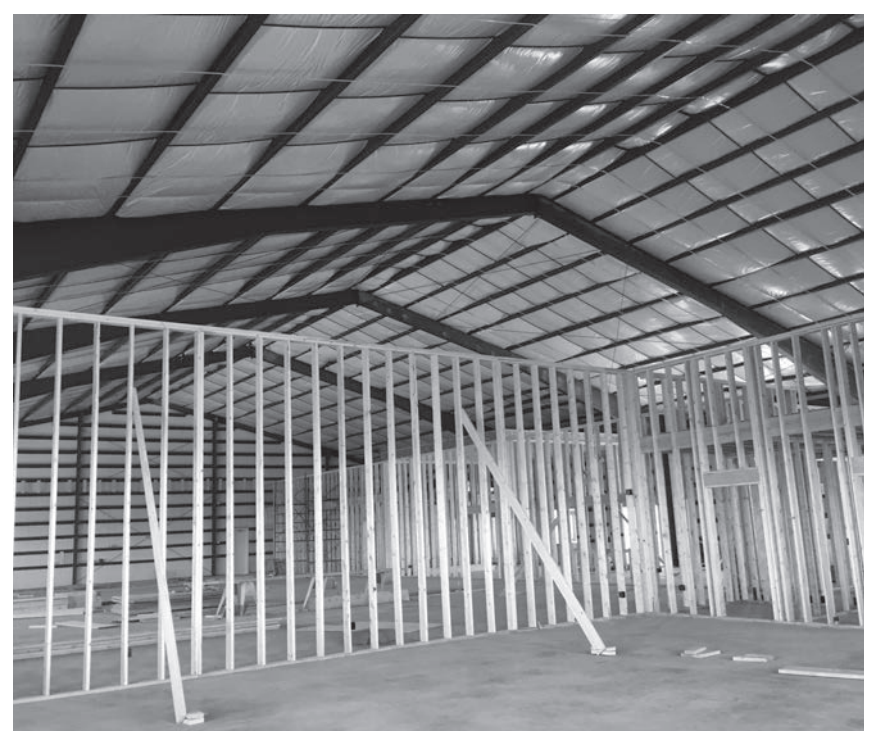
Wall partitions being installed inside of the Tunlii community center.
