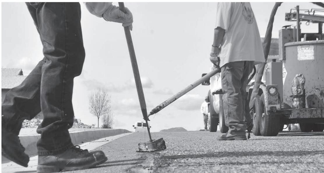
Alvin Stevens (l) levels out the excess tar sealant that Daniel Lewis (back) has applied to the pavement cracks.
