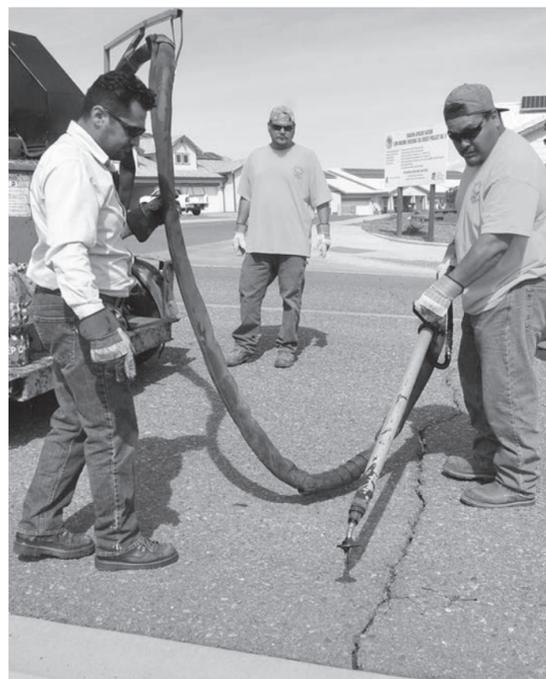
Dexter Beauty under direction of Jason Raya of CRAFCO of Chandler places a sealant in the cracks of the pavement at housing.
